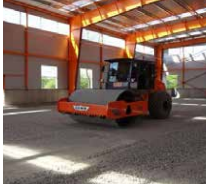
2 Ground Compacting →
