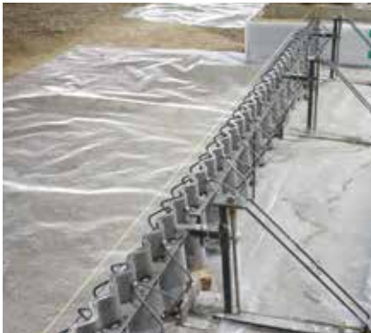
4 Install Construction Joint →
